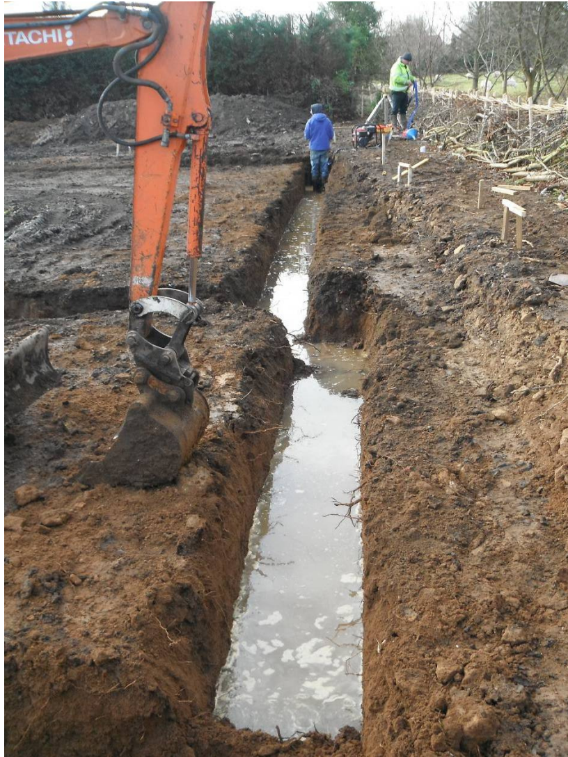
Plate 3: Eastern footings trenches looking south-east.
