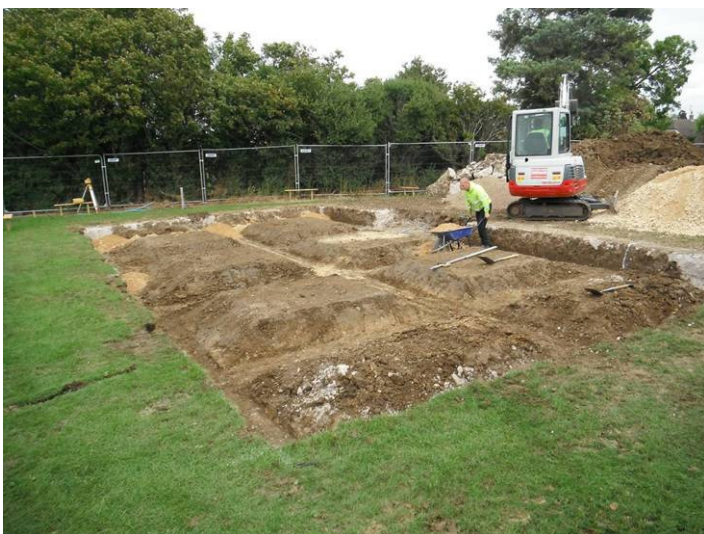
Plate 3: Footing trenches excavated, showing chamfered sides for raft. Looking east.
