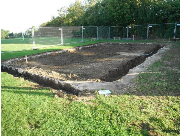
Plate 1: Turf removed and the old concrete footings exposed. Looking north.
