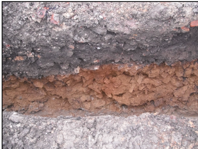
Plate 6: North facing representative section in extension footings to the North of extant building (see Fig 3)
