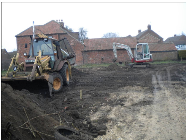
Plate 1: General shot of the site during levelling of Plot 1, looking N.
