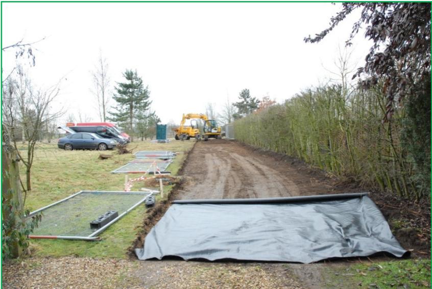
Plate 2: Looking south along stripped access road. Only topsoil (001) exposed.
