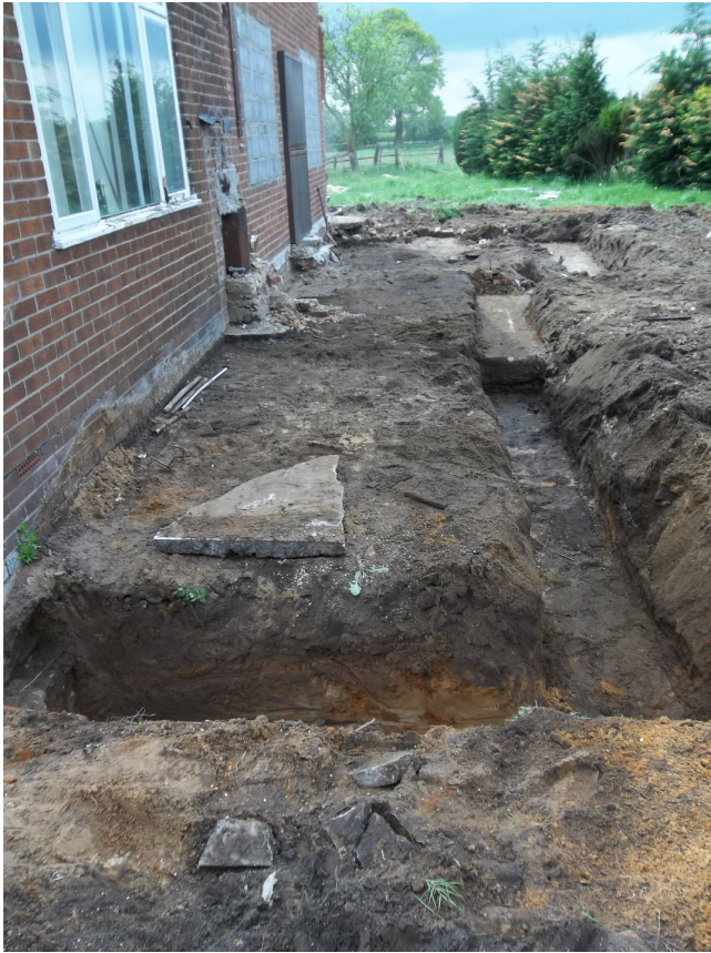
Plate 6: Footings monitored on west side of existing building.
