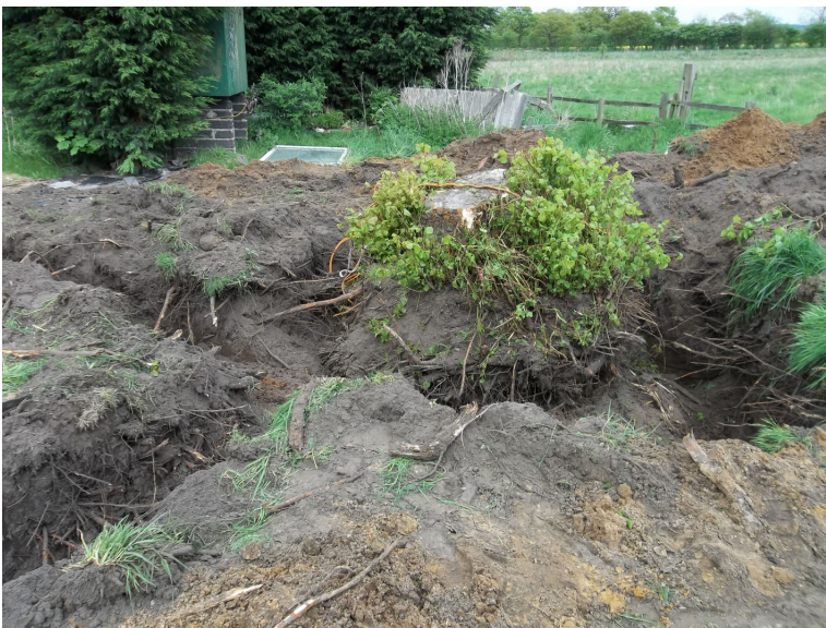
Plate 2: Monitored footings on east side of existing house.
