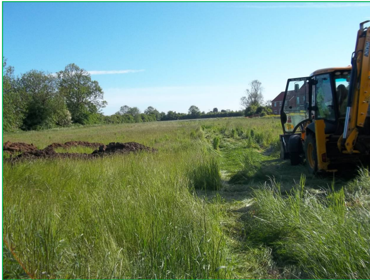
Plate 1: Site shot looking North towards Catchwater Drain
