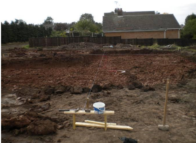
2. Foundation trench for House Plot 6, looking west
