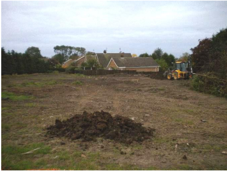
1. The redevelopment site prior to groundworks, looking west
