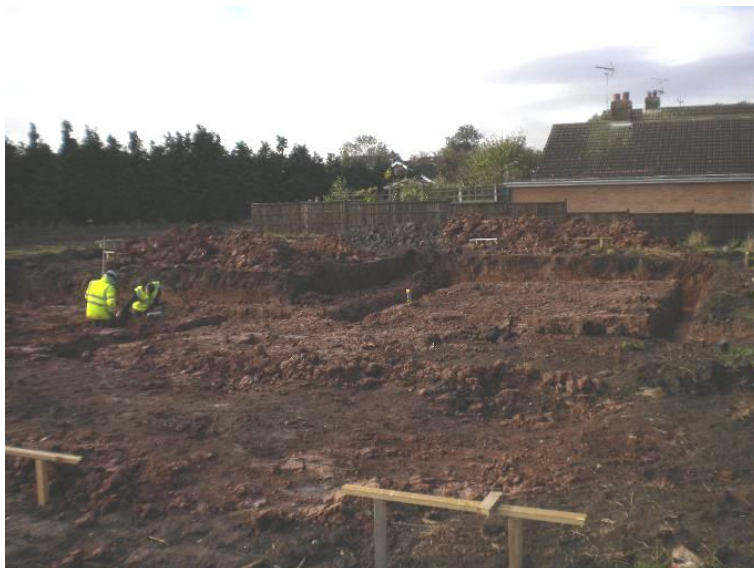
6. Plot 6 fully excavated, looking SW
