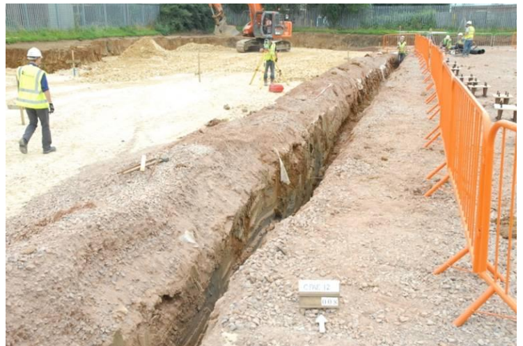
5: Western SEN foundations, looking N
