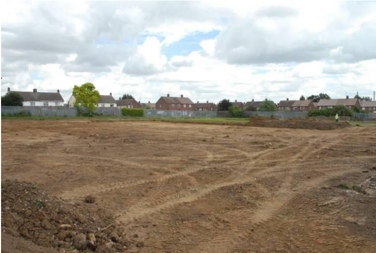
1: Area of SEN building prior to excavation, looking northeast
