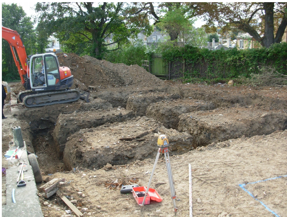
Plate 5: Footings of plot 3 facing north-west
