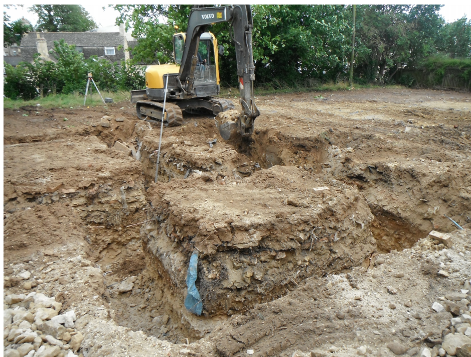
Plate 2: Excavation of made ground facing north-west
