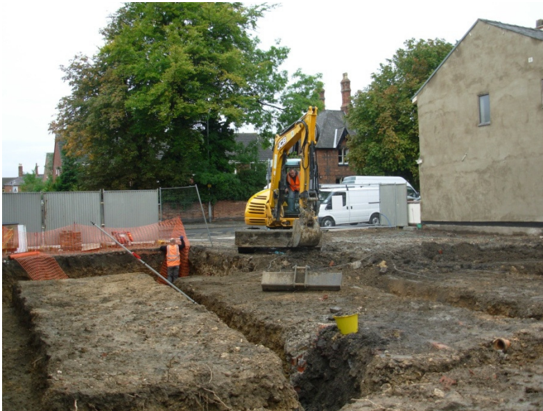
Plate 2: General site shot. Basement [007] in foreground (under yellow bucket).
