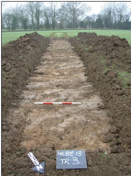
Plate 6: Trench 3 after machining, looking SW towards the S site boundary; no features were encountered in this trench.
