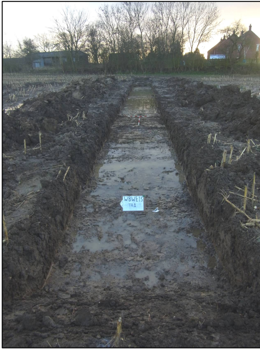
Plate 1: Trench 1 post-excitation, looking SE; the trench is partially flooded.
