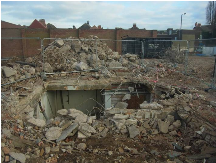
Plate 3: Modern cellar to be backfilled. Looking E
