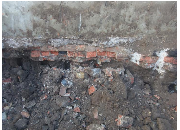
Plate 4: Modern concrete foundations and brickwork overlying 20 th century demolition material. Looking W
