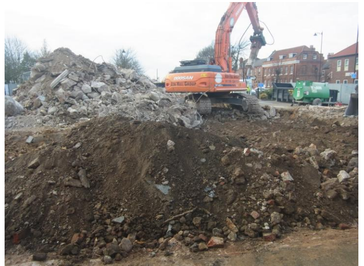
Plate 6: Working shot. Excavated context (002) in foreground. Looking W
