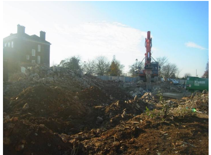
Plate 2: Monitored area. Looking SW
