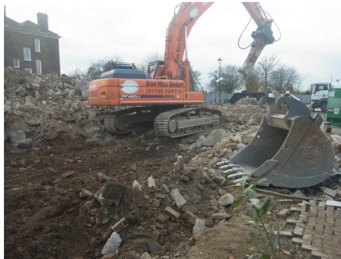
Plate 7: General working shot. Looking SW.
