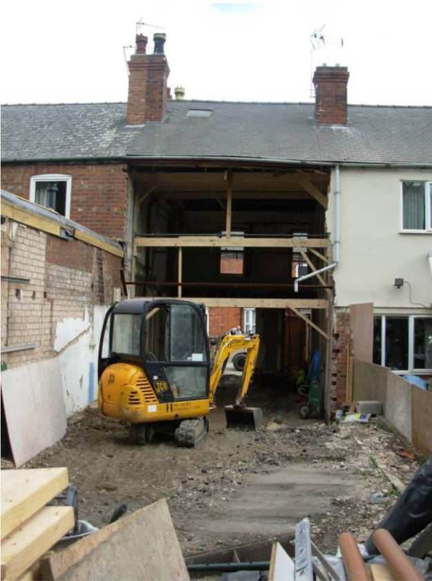
Plate 1: Looking north towards the shell of 37 Cecil Street before excavation commences.
