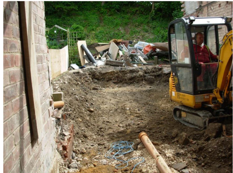
Plate 4: Completed excavations, looking south over reduced ground level.
