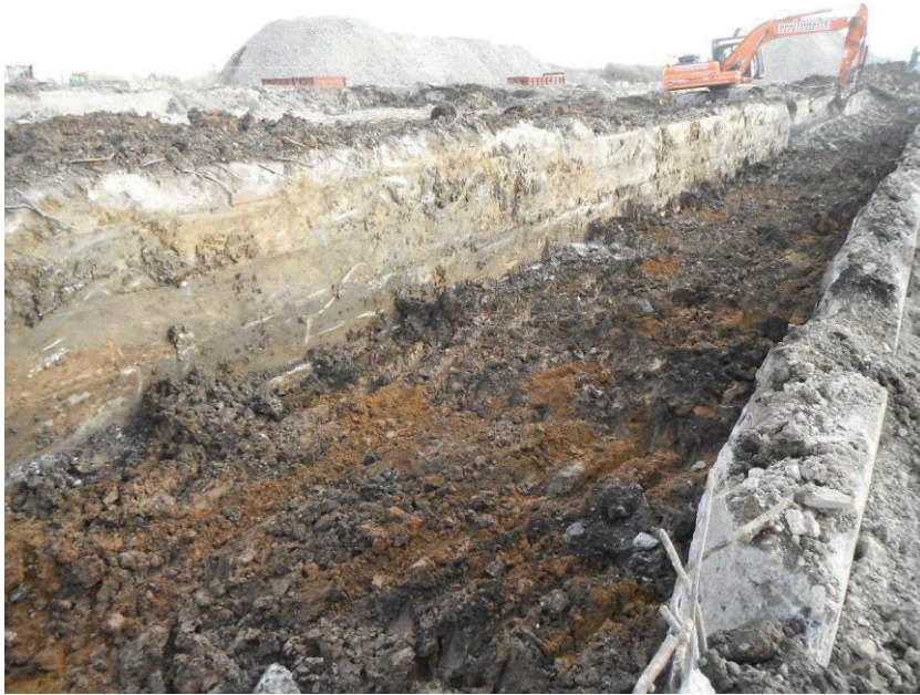
5. Excavation between the remnant concrete footings, looking east
