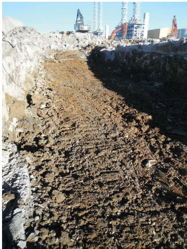
6. View east between remnant concrete footings
