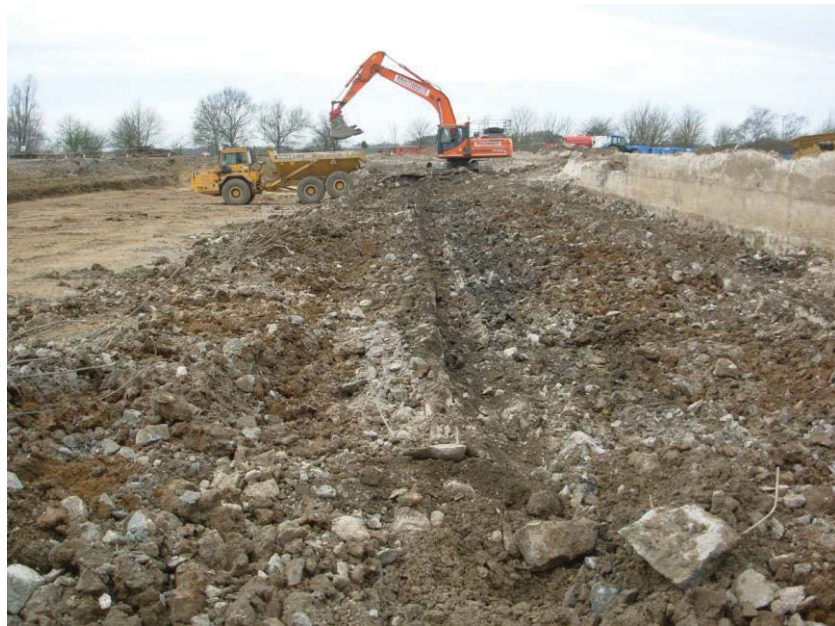
10. View of the north end of the monitoring zone, looking west
