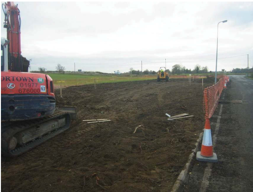
2. Topsoil stripping for the new access road, looking west
