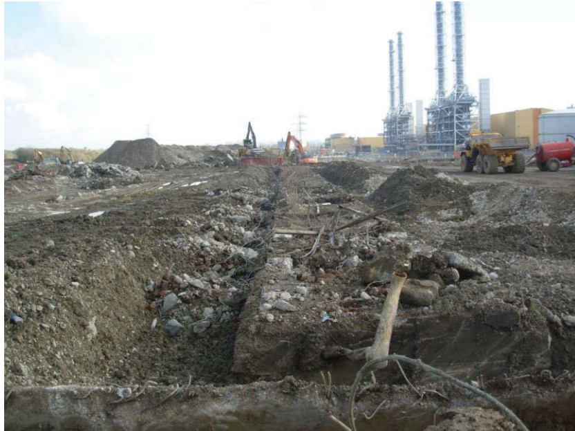
3. The designated monitoring area prior to stripping, looking east
