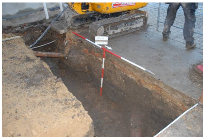
Plate 2: Shot of Trench 2. Looking SW.
