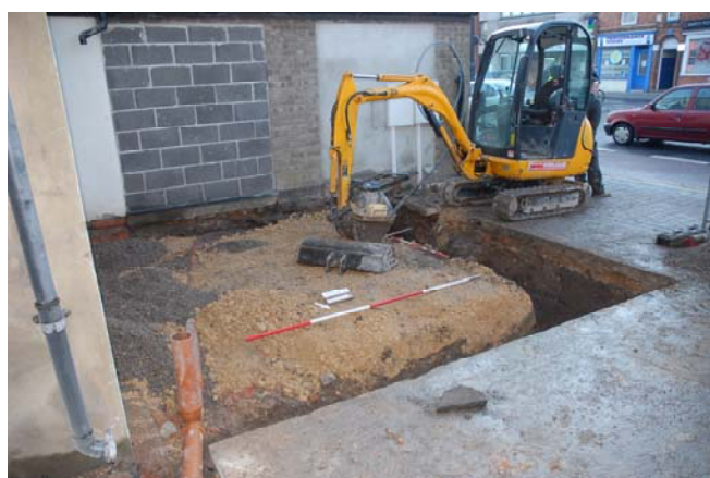
Plate 3: General shot of site. Looking SW.
