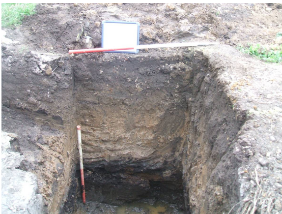
Plate 5: S facing section of Car Dyke [008] (looking N). As with plate 4, (011) can be seen overlying a large peat deposit (010) towards the base of the section.
