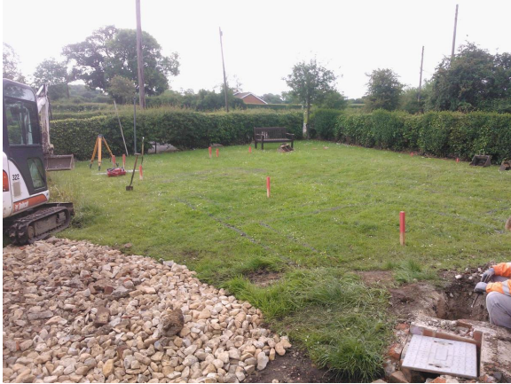
Plate 1: Shot of site prior to groundworks (looking SE).
