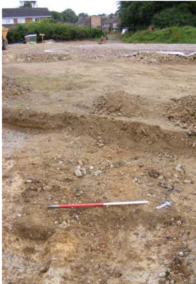
Plate 11: Rough trackway (1106) looking north-west. This ran across the site and was made of hardcore and contained stone fragments and some glassy slag material.
