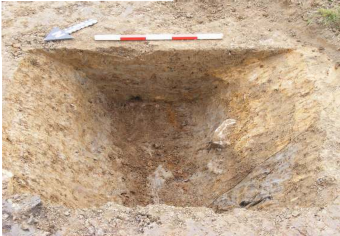
Plate 9: Ditch [1102], looking south-east. A land drain cuts the western edge of the excavated area.
