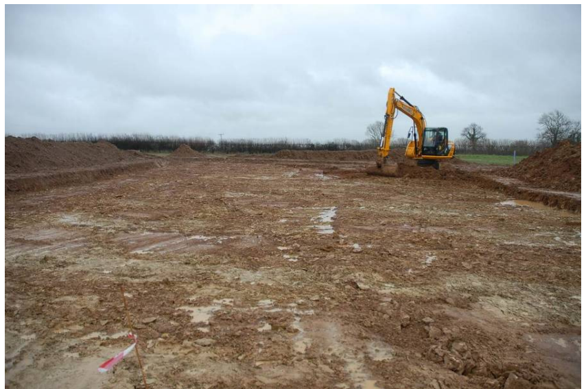
Plate 4: Working shot of excavation of East end of Area 2. Looking E.
