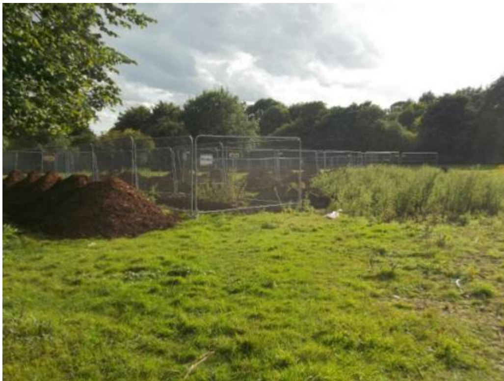
1 General shot of open trenches and erected fencing
