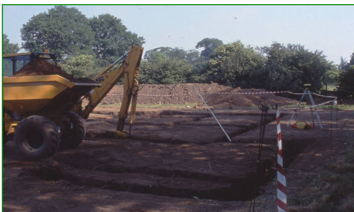
Plate 8 (left): Excavation of the foundation trenches in house plot 7, looking north-west.
