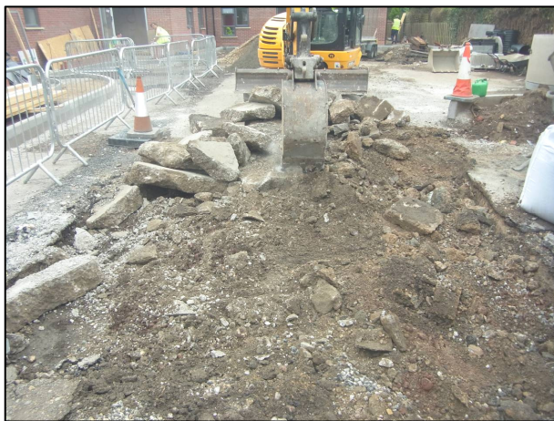
Plate 2: Working shot, looking E across the monitored area, showing the concrete and rubble that required the use of a toothed bucket for machining.
