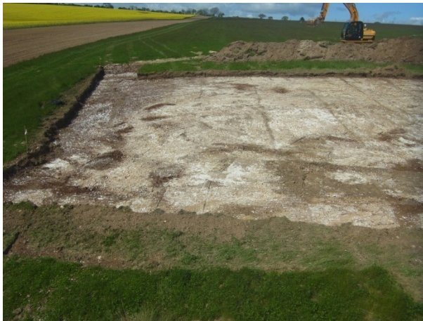
Plate 14: Shot of Area 2 during excavation (looking WNW).
