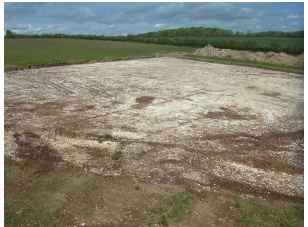
Plate 15: Area 2 excavated (looking NE).
