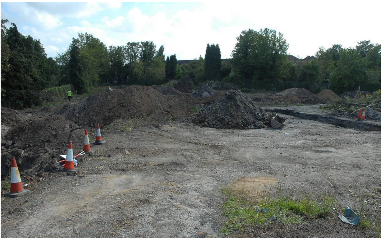
Plate 2: General view of the site, facing SE
