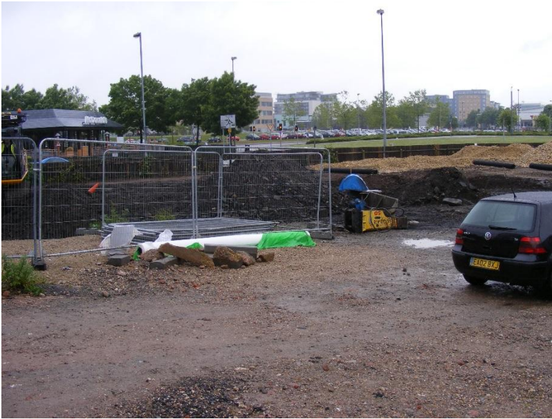
1. Site on arrival on 22/5/14, looking NE
