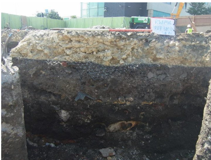
5. Representative Section 2, looking south
