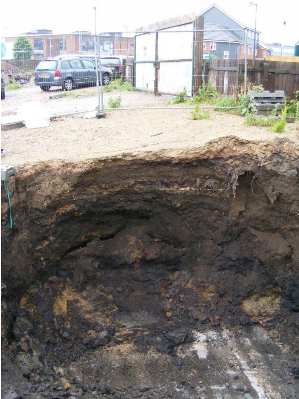
2. Septic tank excavations, looking SW
