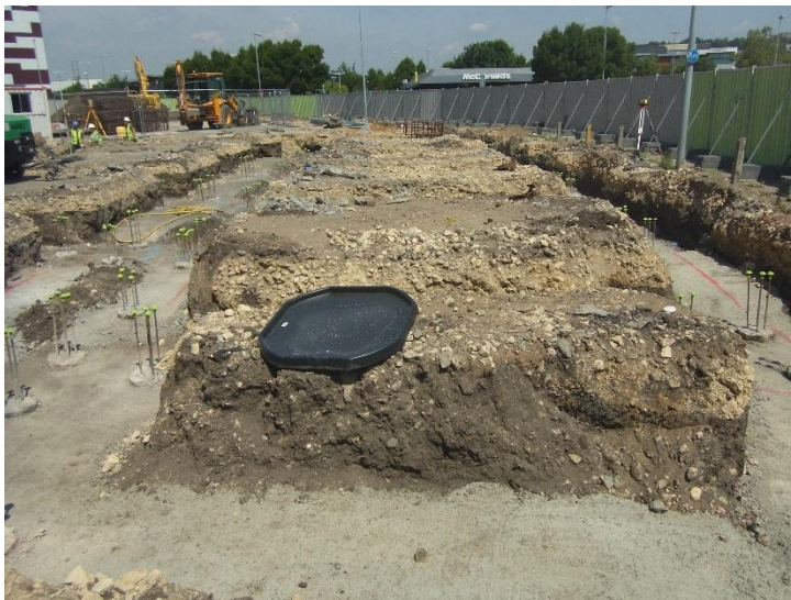
4. General shot of site on 1/7/14, looking north
