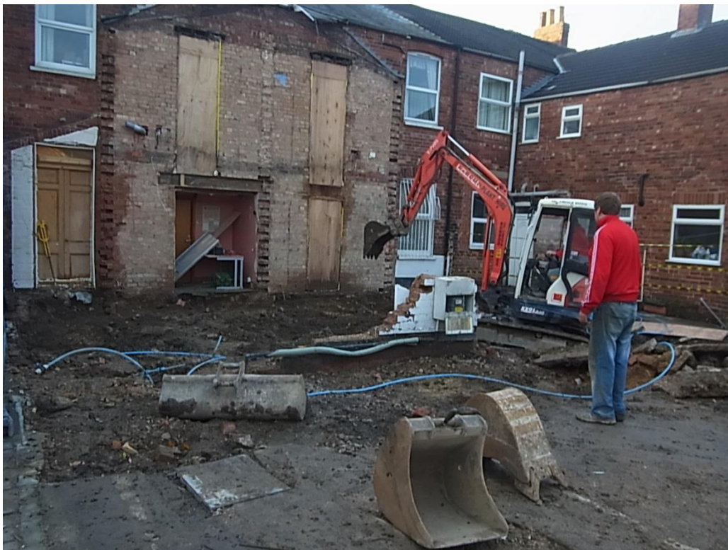
2. General shot of site, looking NW
