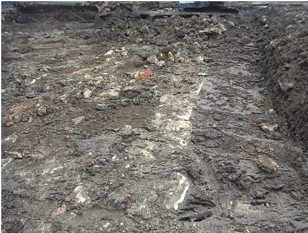
4. Stone footings of demolished structure, looking NW
