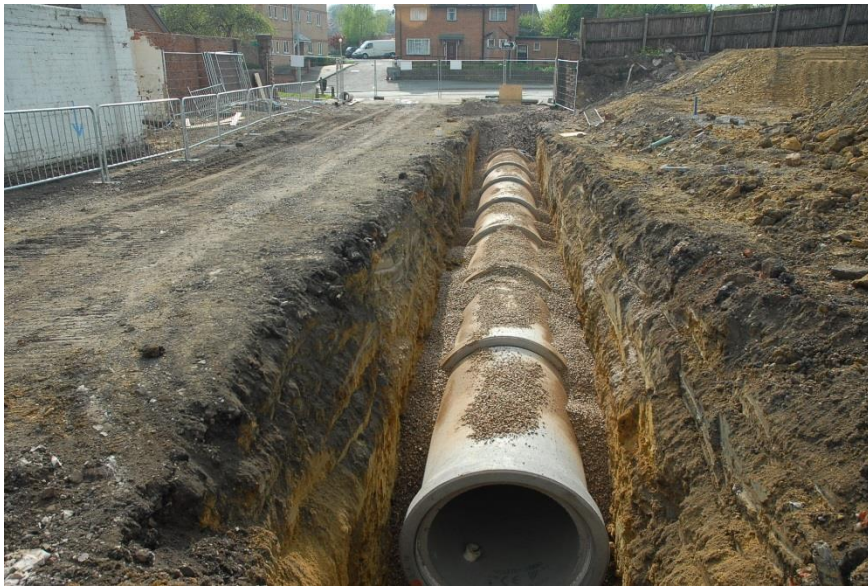
31. General shot of Phase 2 trench, looking west
