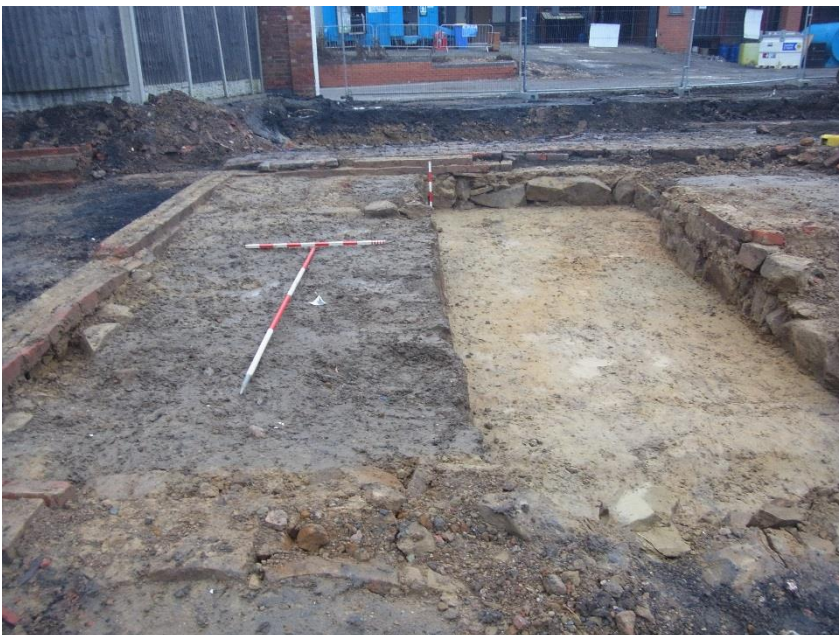
2. Northwest corner of site showing wall 152 (N-S) and pathway 141 (E-W). Looking north.
