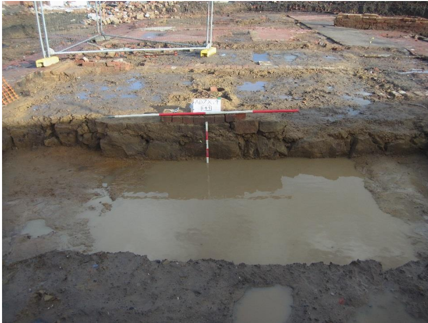
24. Sandstone wall footing 149 and remnants of wall 150, west facing section. Looking east.
