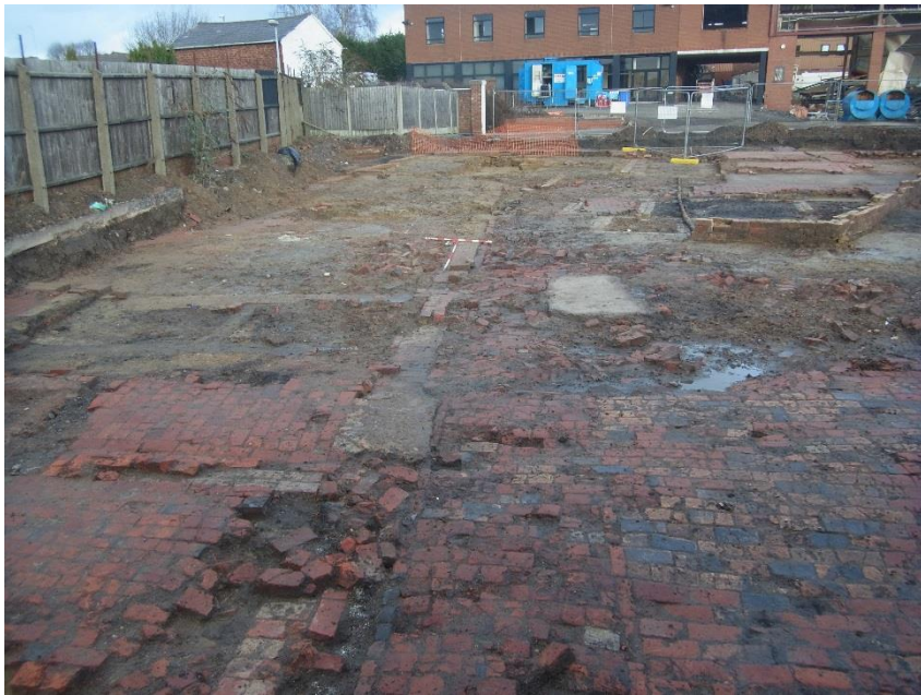
21. General shot of site from southwest corner. Looking north.
