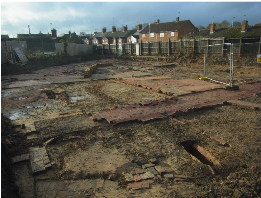
19. General shot of site from northeast corner. Brickwork 146 in left foreground. Looking SW.
