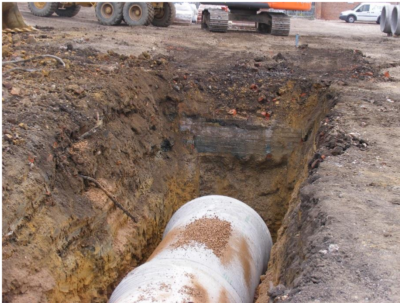
33. Structure 006, looking east
