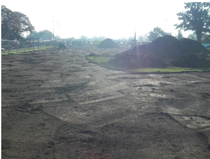
9. Area 2. Site on arrival, looking east
