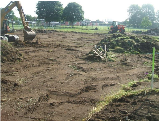
1. Area 1. Site on arrival, looking NE
