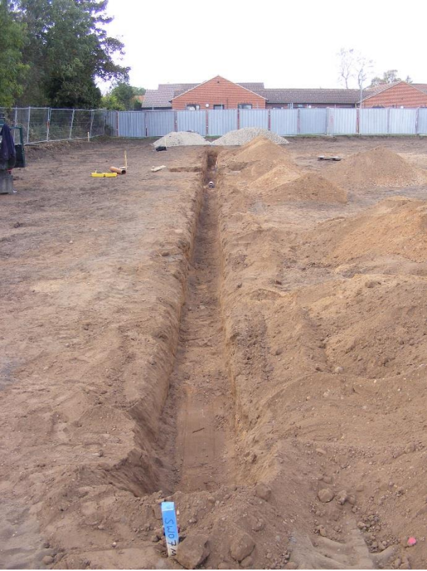
13. General shot of shallow trench, looking west
