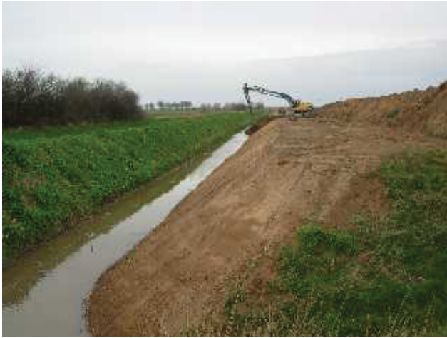
Plate 1: The drain being widened. This view was from a footbridge, but the monitoring took place from the opposite bank
