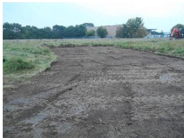
Plate 2: Excavation of Area 1 (looking south-east).
