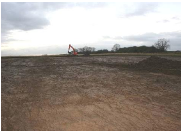
Plate 12: Excavation of Area 4 (looking south-west).
