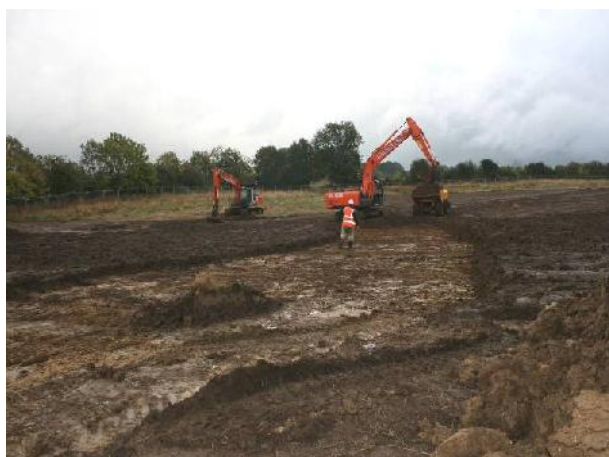
Plate 3: Excavation of Area 2 (looking north).
