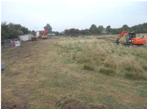
Plate 1: Excavation of Area 1 (looking north).
