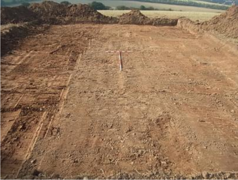
Plate 4: Area 2 looking North
