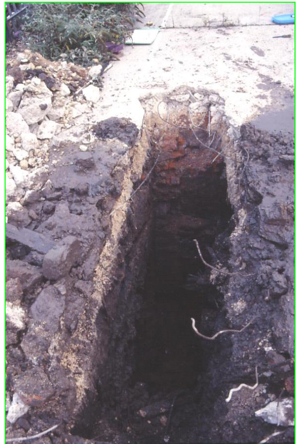
Plate 4: Test Pit 2, looking south
