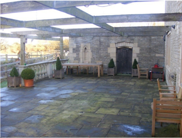
Plate 1 – Patio area prior to excavation (looking north).
