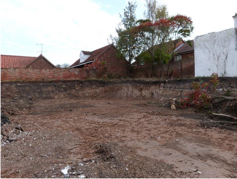
9. Completed excavations of ground reduction area, looking northeast
