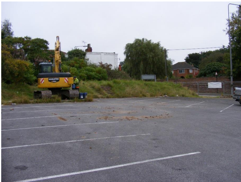
2. Pre-excitation shot of site, looking southeast
