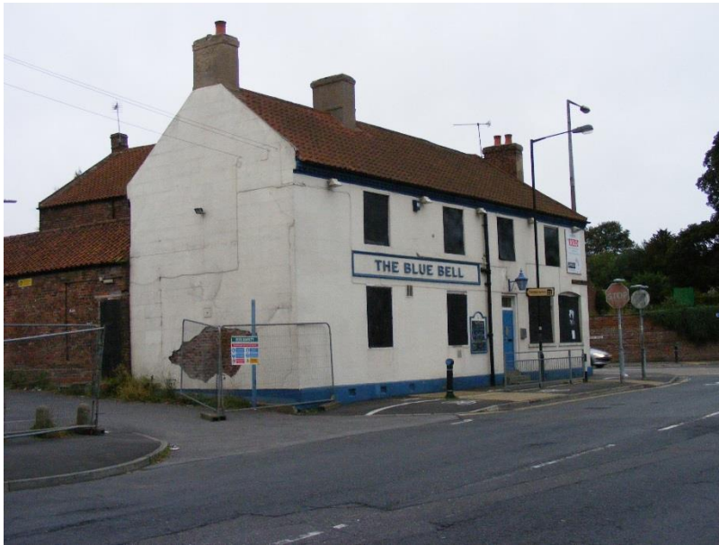
1. The Blue Bell, looking southeast
