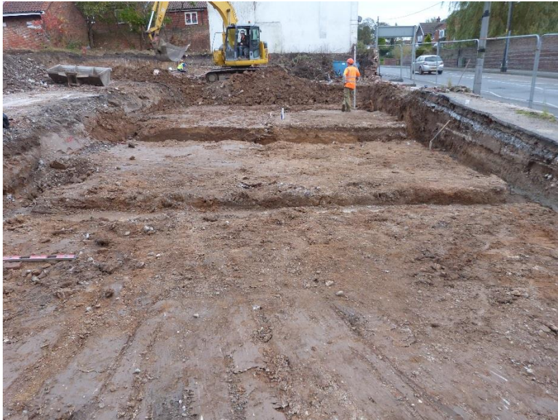
15. Completed footings excavation, looking east
