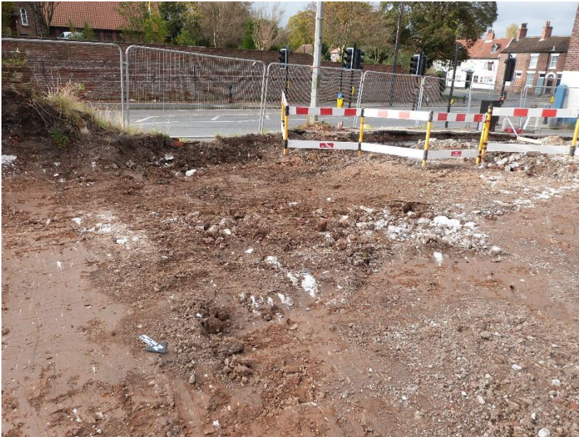
10. Overview of construction cut [111] and robbed out wall 108, looking southwest
