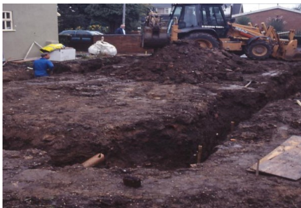
Plate 2: Foundation trenches looking east.
