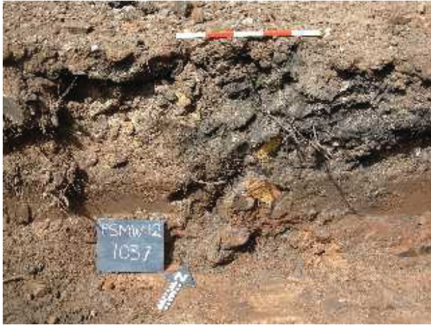
Plate 10: Foundation of sandstone wall (1037) looking north. It is probably the Foundations of the current boundary wall to the rear of Plot 9.
