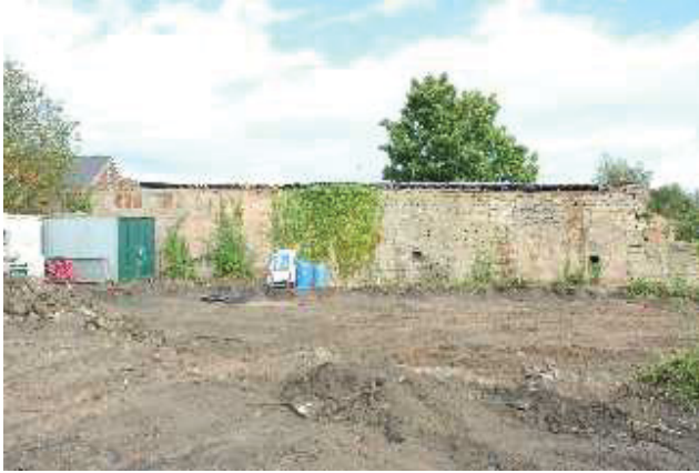
Plate 1: Outbuildings as viewed from the south-west. These were lace-making cottages during the 19 th century. Boundary wall (1004) is on the far right of the photograph.
