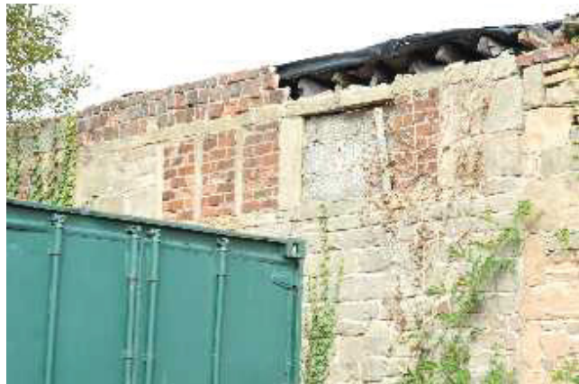
Plate 2: Windows of the outbuildings. Situated on the first floor, the long styled windows were characteristic of lace-making cottages in Nottinghamshire.
