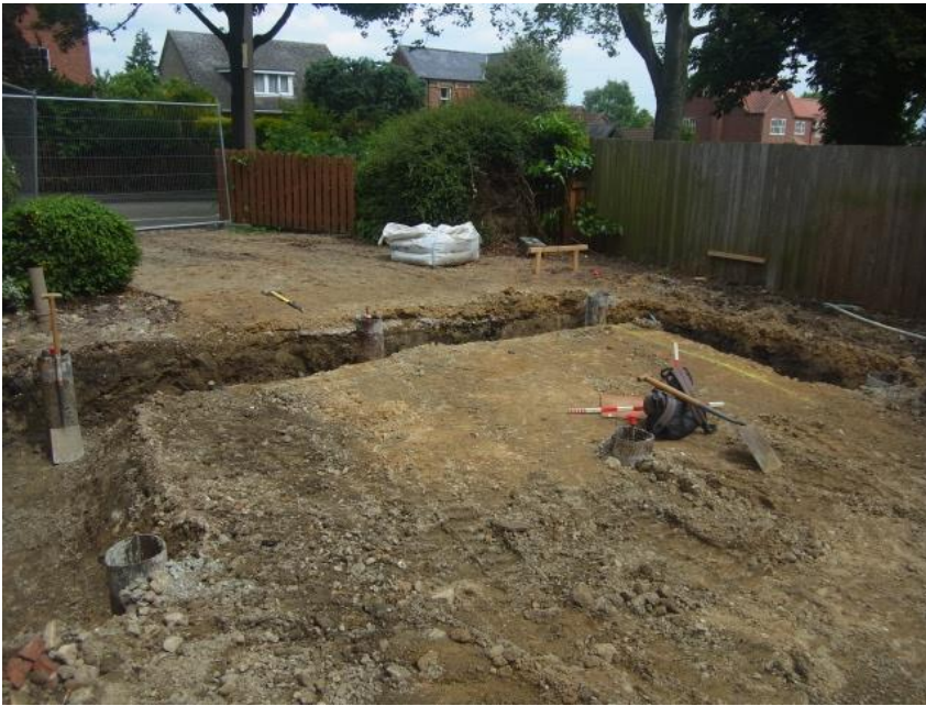
1. Site on arrival, looking northeast. (Excavations began without monitoring)
