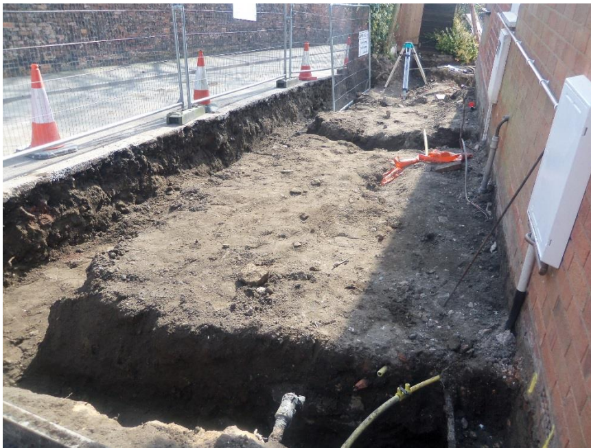
8. Completed excavations, looking south
