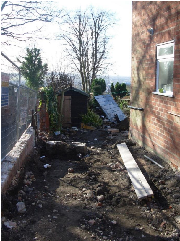
1. General shot of site on arrival, looking south
