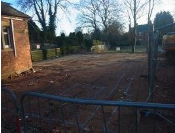
PL. 1: General view of development area with footings marked out.
