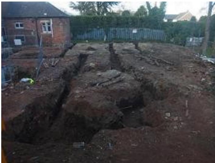
PL. 2: General view of footing trenches facing north
