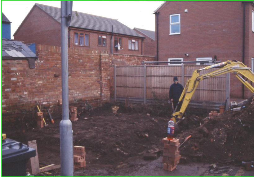
Plate 4: Completed foundation excavation, looking northeast
