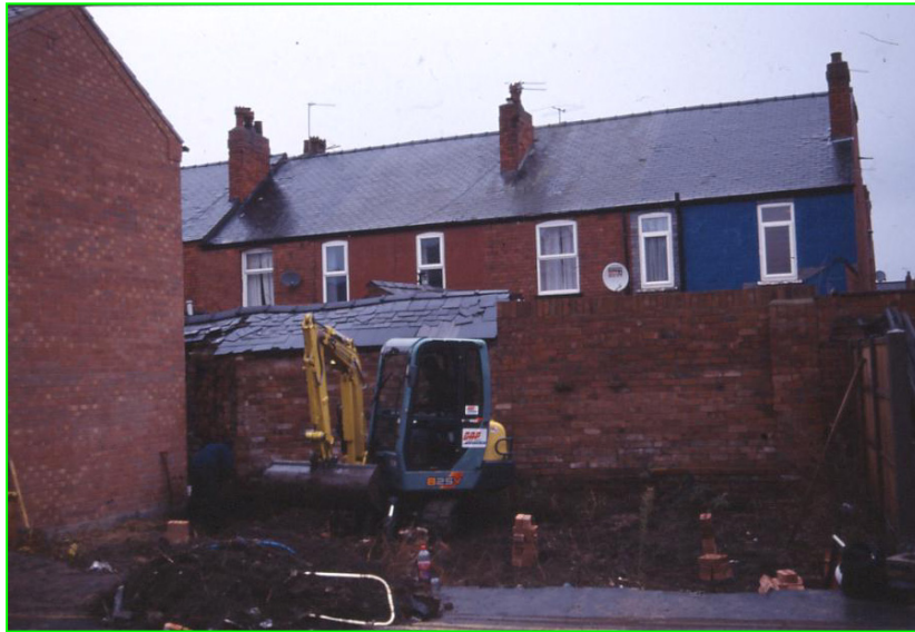
Plate 1: Work in progress, looking north
