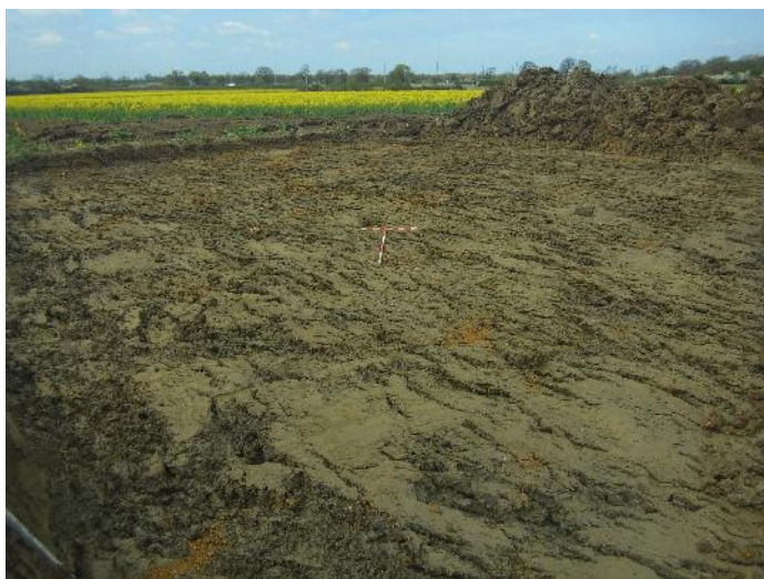
Plate 2: The south-west end of the crane pad onto natural clay
