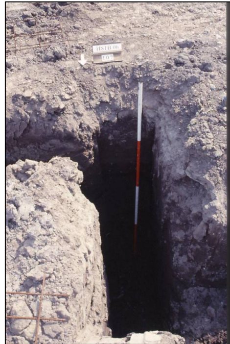
Plate 5 (above): Stanchion pit [107], looking south.
