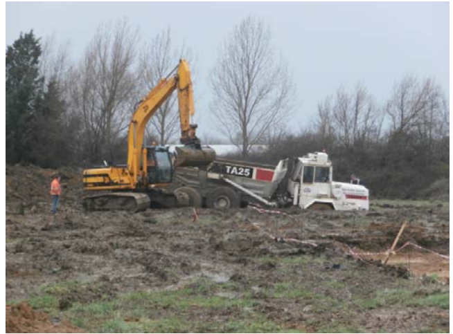
56. Area B working shot looking NW
