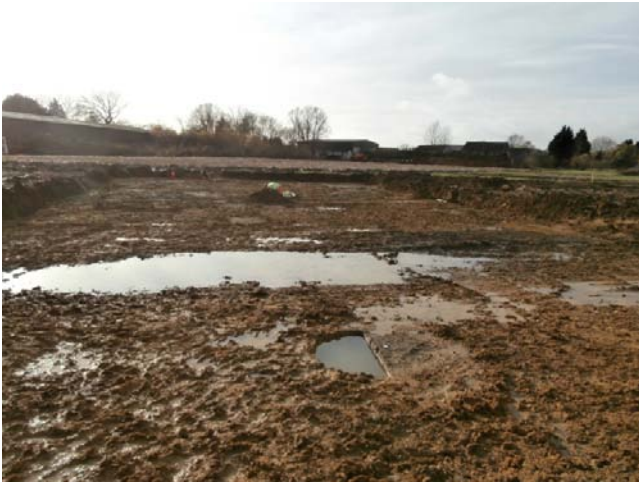
21. Area B working shot looking SW
