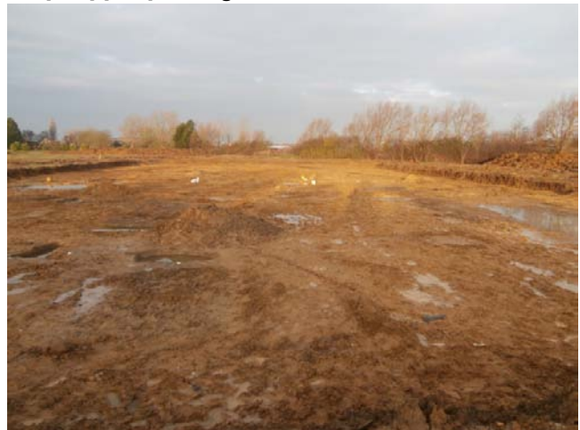
40. Area B working shot looking NW
