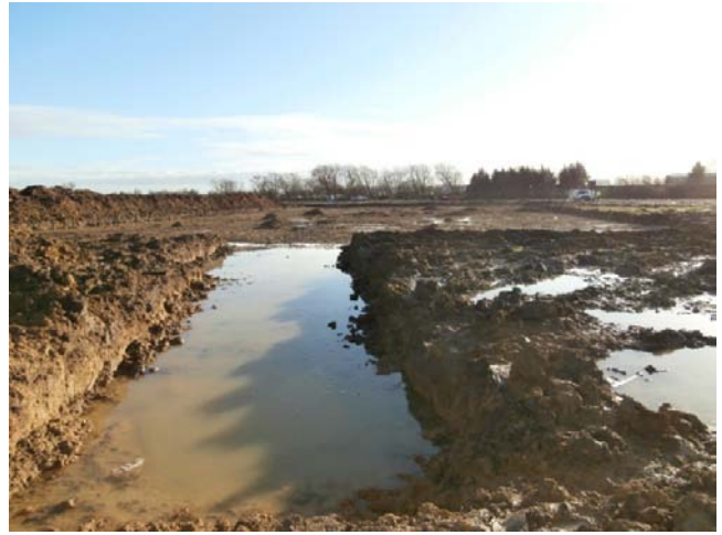
80. Area B post-excavation looking SE
