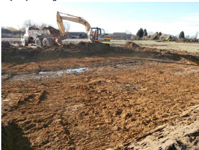
11. Area B working shot looking SW
