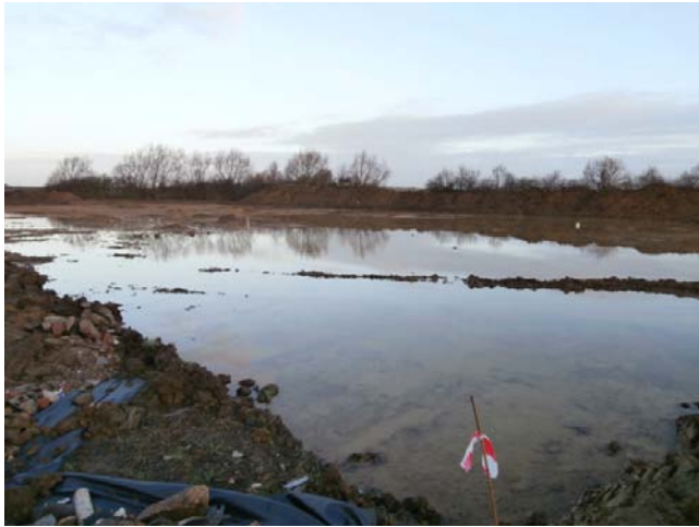
63. Area B working shot looking NW
