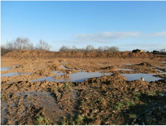
79. Area B post-excavation looking NE
