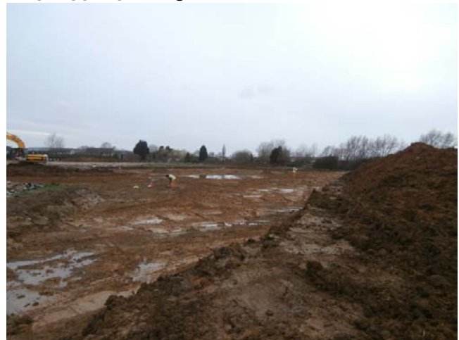
54. Area B working shot looking W
