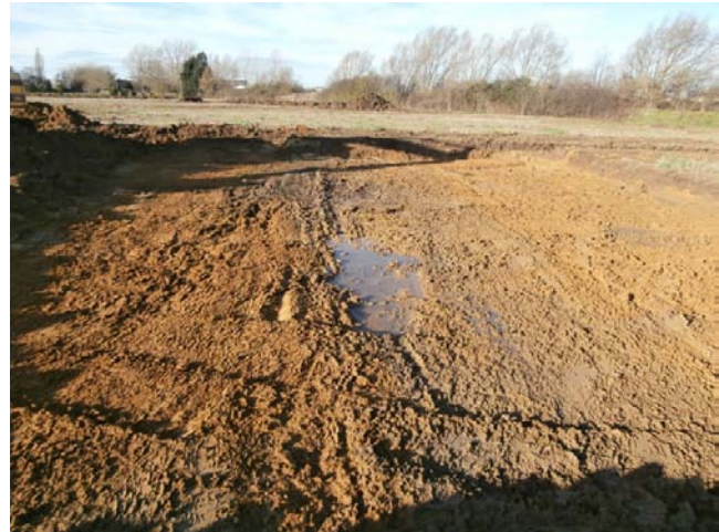
10. Area B working shot looking NW
