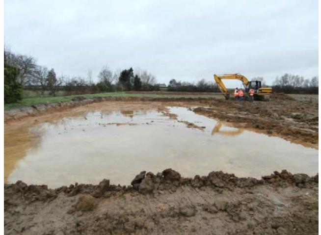
2. Area A working shot looking N
