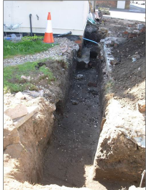
Plate: 2. Excavated footings on east side of development, looking south.
