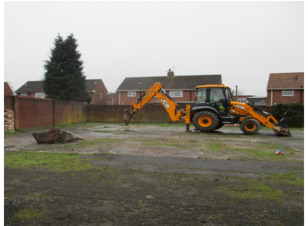
Plate 2: Pre-excitation shot of area where Trench 1 was positioned (looking SW).
