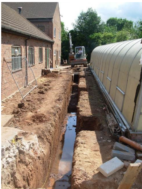
Plate 4: Partly excavated foundation trenches, looking east
