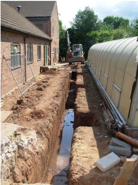
Plate 4: Partly excavated foundation trenches, looking east
