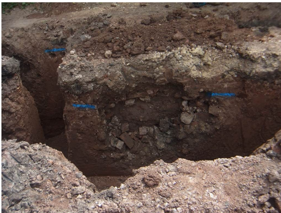
Plate 7: West facing section showing soakaway feature [112].
