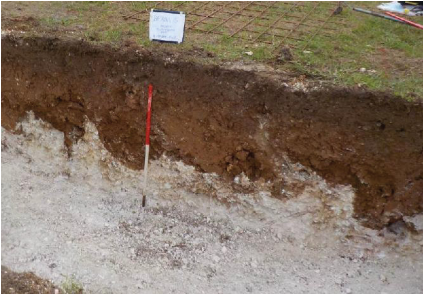
Section of Foundation Trench for "Private Switchgear" – Looking East
