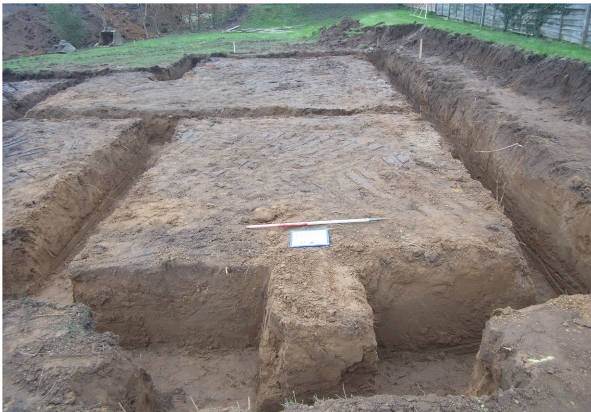
Plate 2: General shot foundation trench post excavation, looking south-east
