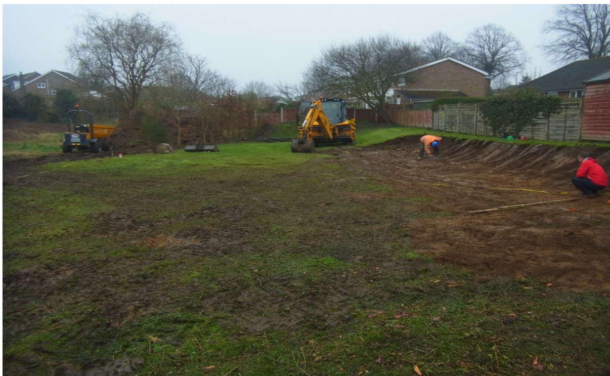
Plate 1: General shot of initial groundworks, looking south-east
