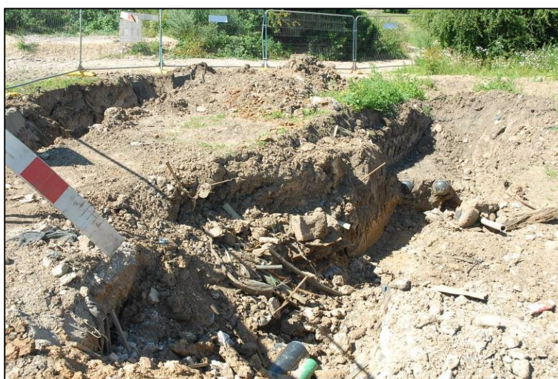
Plate 5: Modern demolition material in Excavation 5
